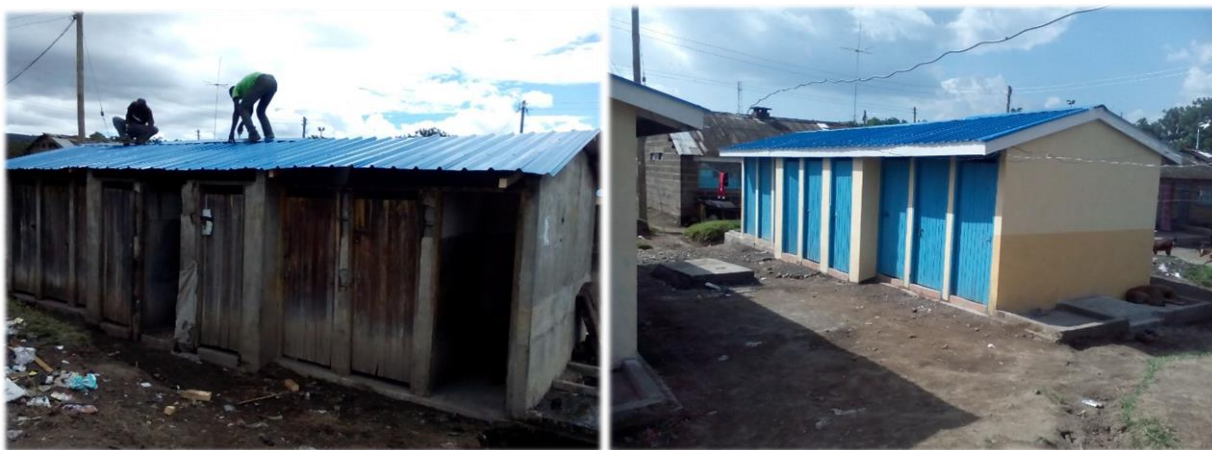
Plate 3.1: County Estates' face-lifting in Kimathi
