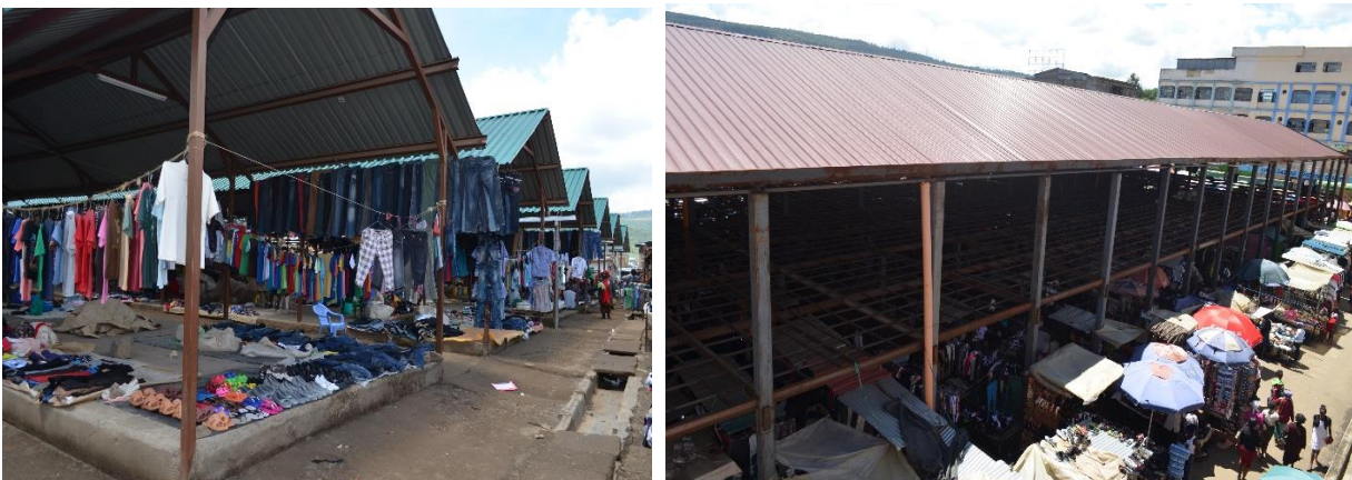
Plate 3.6: Constructed Market Sheds in Mai Mahiu and Nashar
