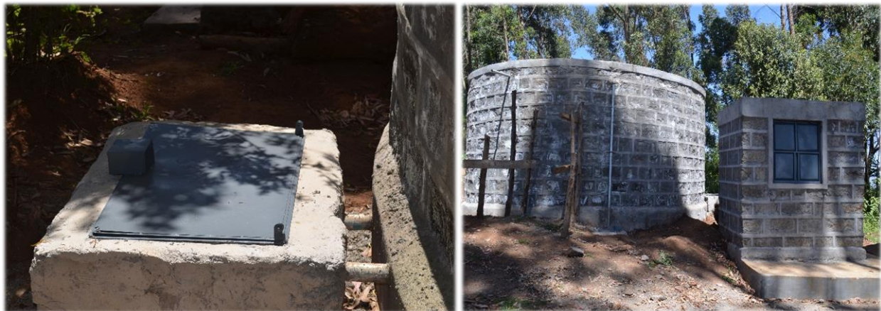
Plate 3.7: Water Project in Kuresoi North
