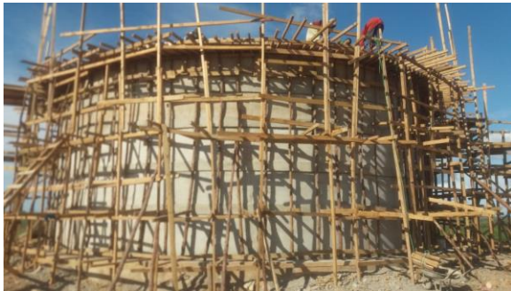
Figure 1: Concrete tank under construction
