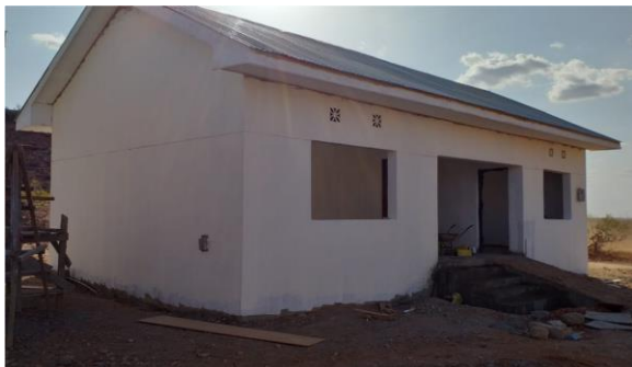
Figure 2: IUWA office under Construction
